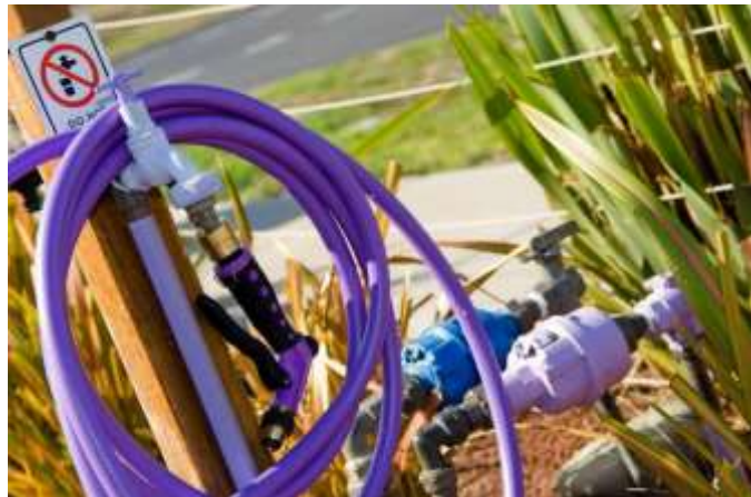
Figure 19 Non potable water reuse (recycled water) infrastructure at household
